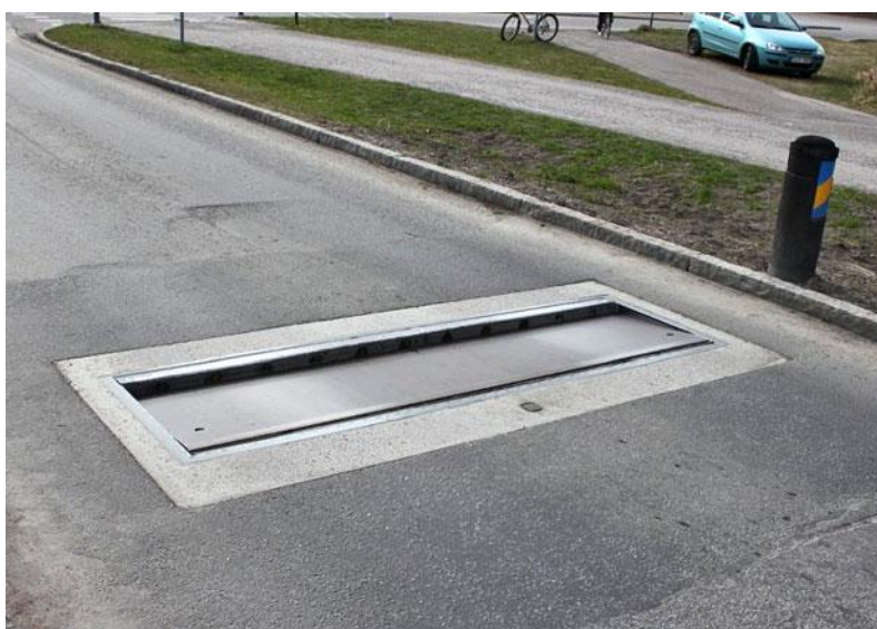
Fig. 2. Active speed bump [2]
